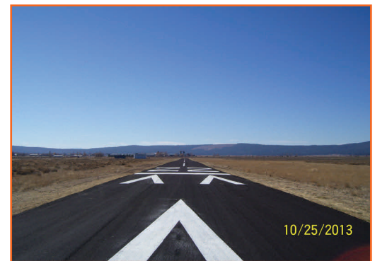
Runway After Construction
