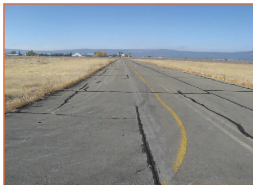
Runway Before Construction
